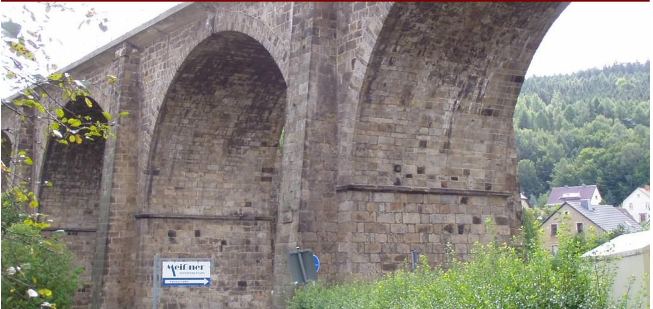
Rich natural resources of granite were used in the construction of the railroad bridge on the railroad line Dresden-Görlitz.
